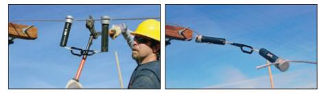
2. Safely cut slack conductors (up to 200 lbs. of tension between Clamp & Carabiner) while maintaining positive control of loose ends.
